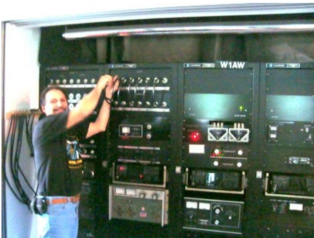
Setting up the antenna patches
