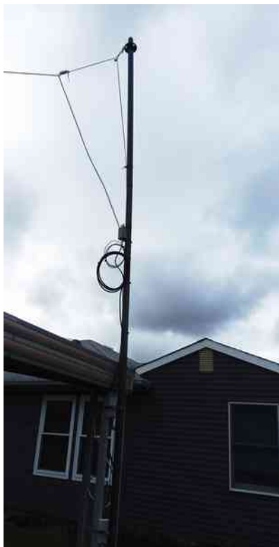
At first, the antenna was run around the side of the house, touching the roof.
