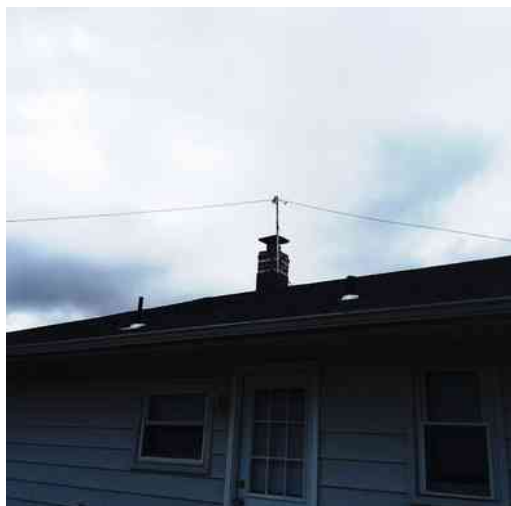
A chimney mount with a five-foot pole was added to carry the antenna over the roof.
