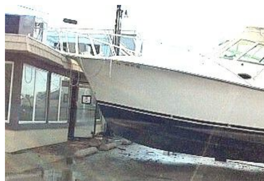
Boat resting on Taylor's Restaurant in Point Pleasant Borough after Hurricane Sandy. Photo by Carl LeFevre. WA2IQE
